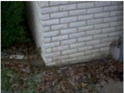
Soil should be a minimum of 4" below foundation all around house to prevent water intrusion and insect infestation.
