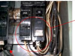
These 2 breakers are not designed for two wire usage. Only one screw is present on each breaker. Recommend electrical specialist to evaluate and repair as needed.
